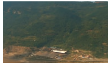
Three Gorges Hydropower Complex
