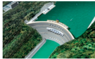
Xiluodu Hydropower Plant (under construction)
