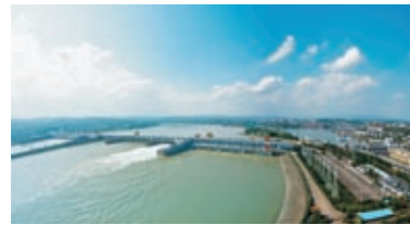
Gezhouba Hydropower Plant
