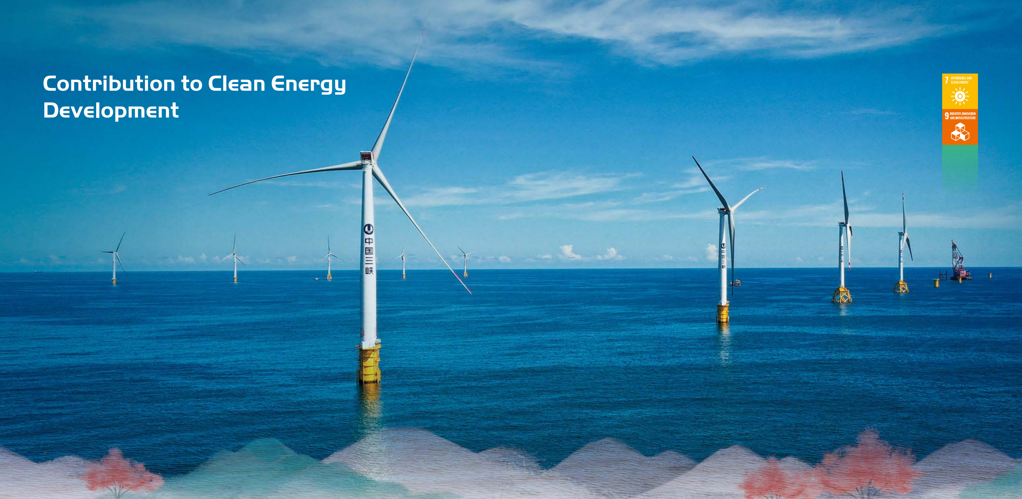
Yangjiang Offshore Wind Farm in Guangdong Province
