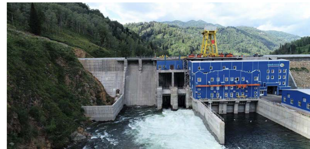
Turguson Hydropower Station in Kazakhstan
