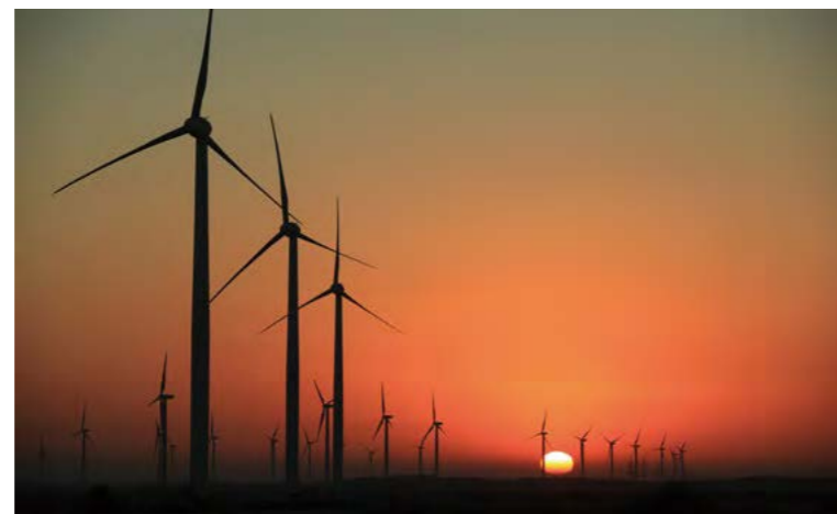
The Three Gorges First Phase Wind Power Project in Pakistan
