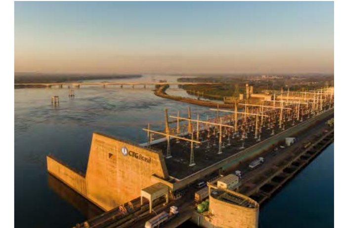
The Jupia Hydropower Plant
