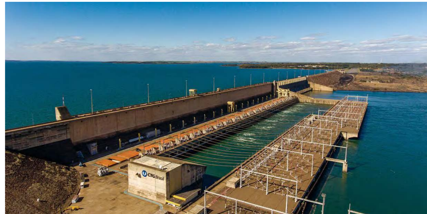
The Ilha Solteira Hydropower Plant
